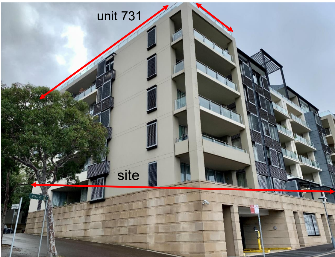
Figure 4: Building E (site) viewed from corner of Bayview Street and Mill Street
